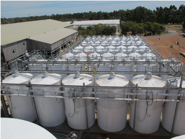
Modern tank farm in Western Australia
